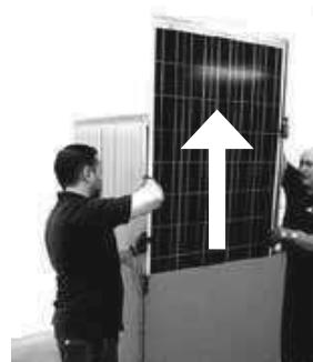
4 Remove the upper cardboard box by directly lifting it upwards. (Two people are necessary!)
